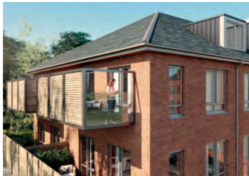
Balconies to apartments 4, 5, 7 & 8
